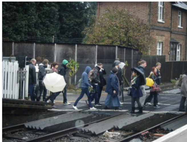
Figure 4 – View of the crossing looking south from the western platform
